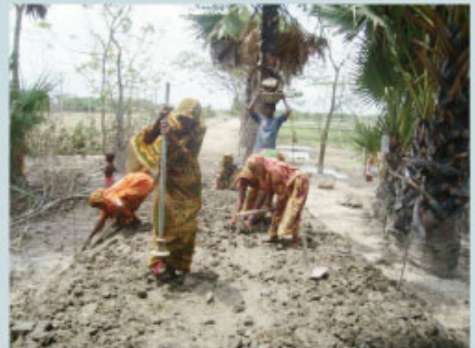
Community Infrastructure Works are going on.
